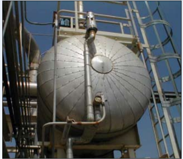
AL6XN constructed Brine Storage Tank for local co-gen facility
